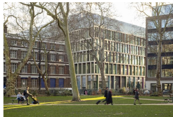
Kaleidoscope Building (OSD) over Farringdon East Crossrail Station: OSD completed Dec 2019.
